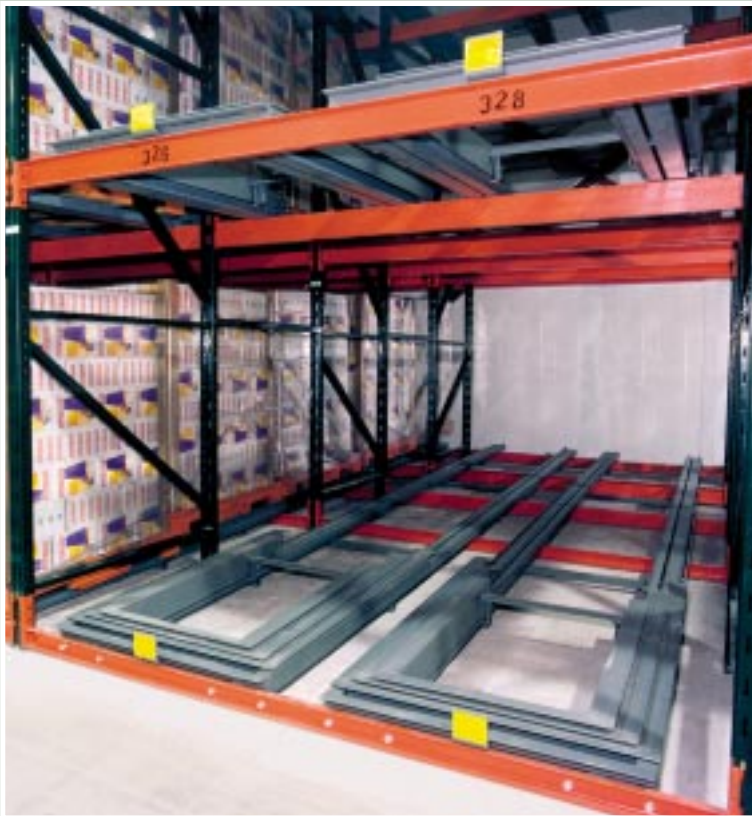
▲ 5 deep pushback floor mounted
